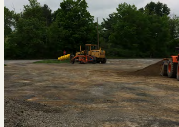
Looking out from the shed to CR 27
